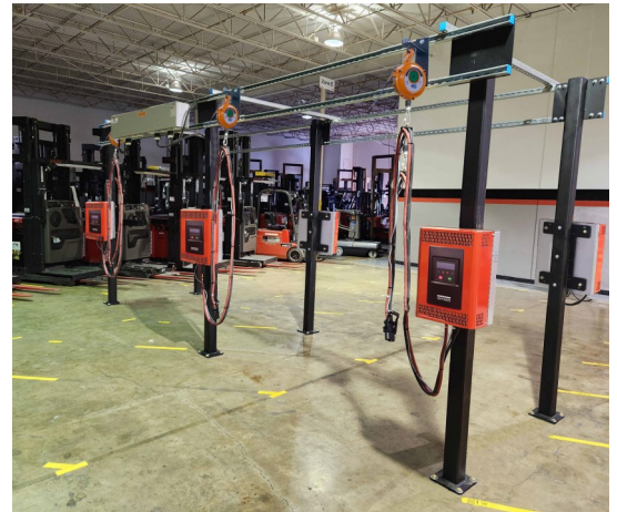
CSHFM-0001 Installed in Series w/Hanging Cable Balancer, BCR-H5-KIT
