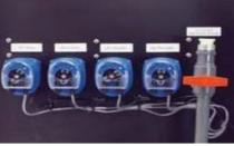
The MWTS utilizes four chemicals: Sodium Hydroxide, (Caustic), MetalEX, Aluminum Sulfate (Alum sed as a Coagulant) and Polymer. Adustable speed chemical injection pumps are used for injecting chemicals into the treatment tank
