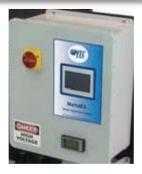
The MWTS is controlled by the PLC. The PLC monitors liquid levels, pressure, flow and adjusts accordingly.
