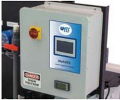
The MWTS is controlled by the PLC. The PLC monitors liquid levels, pressure and flow and adjusts accordingly.
