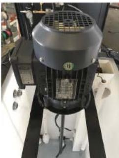
The paddle mixer in the treatment tank turns on when the top liquid level sensor in the treatment tank has lifted. The mixer motor speed is controlled by a VFD (Variable Frequency Drive) and is preset to 25 Hz.
