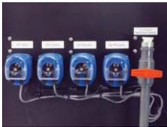
The MWTS uses four chemicals: sodium hydroxide, (caustic,) MetalEX, aluminum sulfate (alum used as a coagulant) and polymer. Adjustable speed chemical injection pumps are used for injecting chemicals into the treatment tank.
