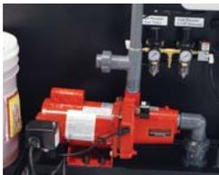
The MWTS recycle system includes a pressure pump that is set to turn off at pressure above 50 PSI and turn on at lower pressure. Pumps are fully automated and do not require a pressure tank to maintain pressure.
