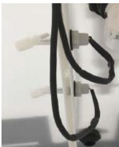
Liquid Level Sensors: Reed type liquid level sensors are used throughout the system to monitor the water levels in the tanks. Liquid level sensors control the flow of water into and out of the surge tank.
